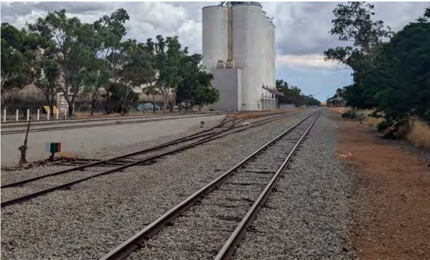
Figure 14 Existing Surrounding Landscape Character - Railway Track
