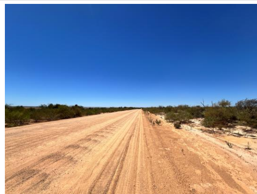
F17.4: Gate 12 Approach Looking Right (North)
