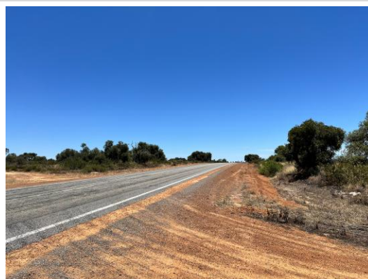
F9.4: Gate 4 Approach Looking Right (Southwest)
