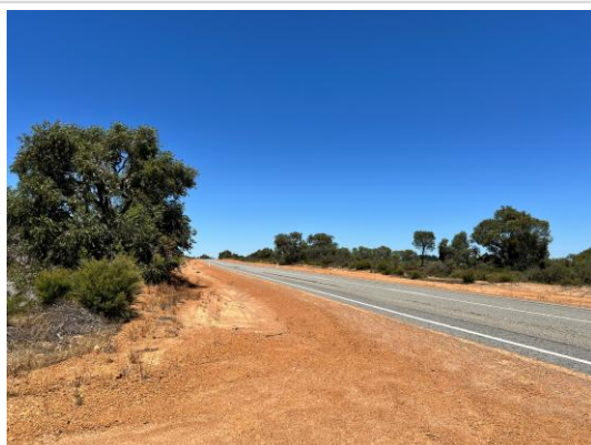
F7.3: Gate 2 Approach Looking Left (Southwest)
