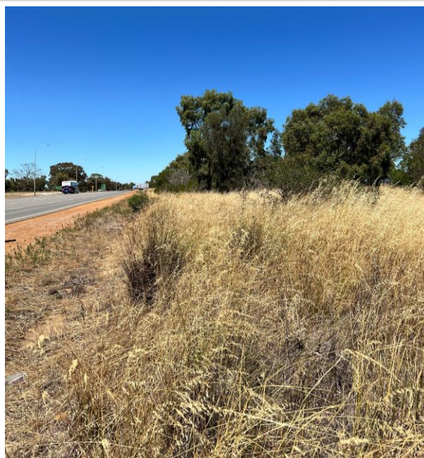
F1.10: Brand Highway Facing South from Western Verge
