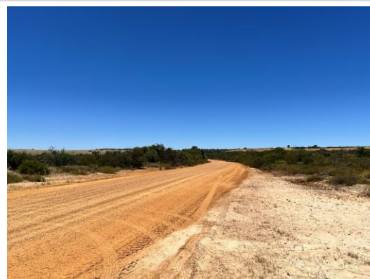
F14.4: Gate 9 Approach Looking Right (East)
