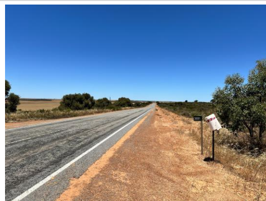
F19.4: Gate 14 Approach Looking Right (Southeast)
