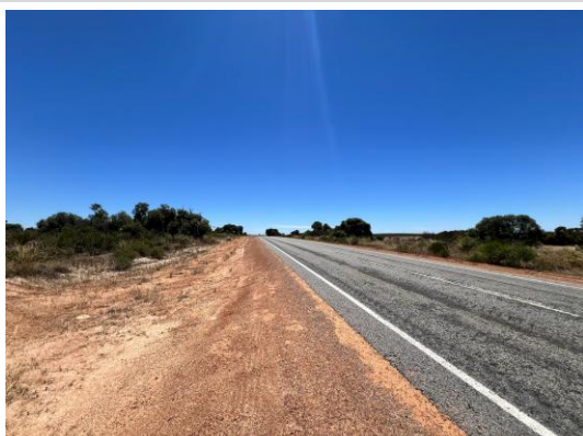
F19.3: Gate 14 Approach Looking Left (Northwest)
