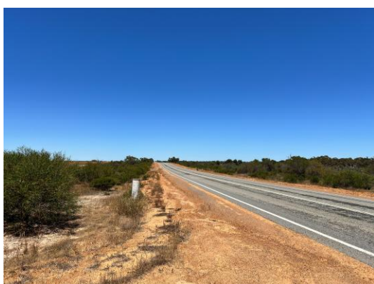
F20.3: Gate 15 Approach Looking Left (Southwest)
