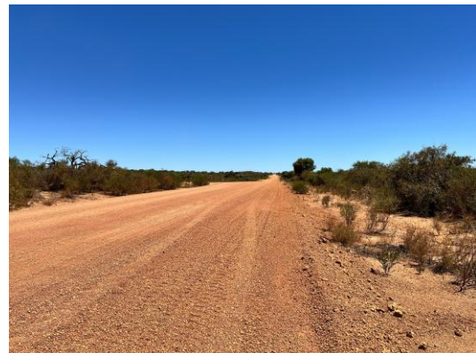
F16.4: Gate 11 Approach Looking Right (South)
