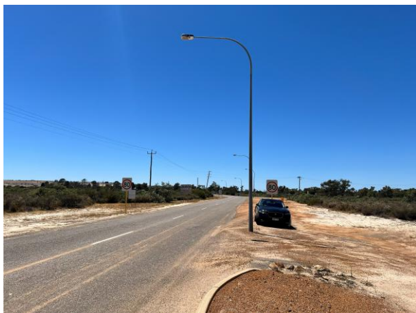
F1.7: Three Springs-Eneabba Road Facing East from Southern Verge
