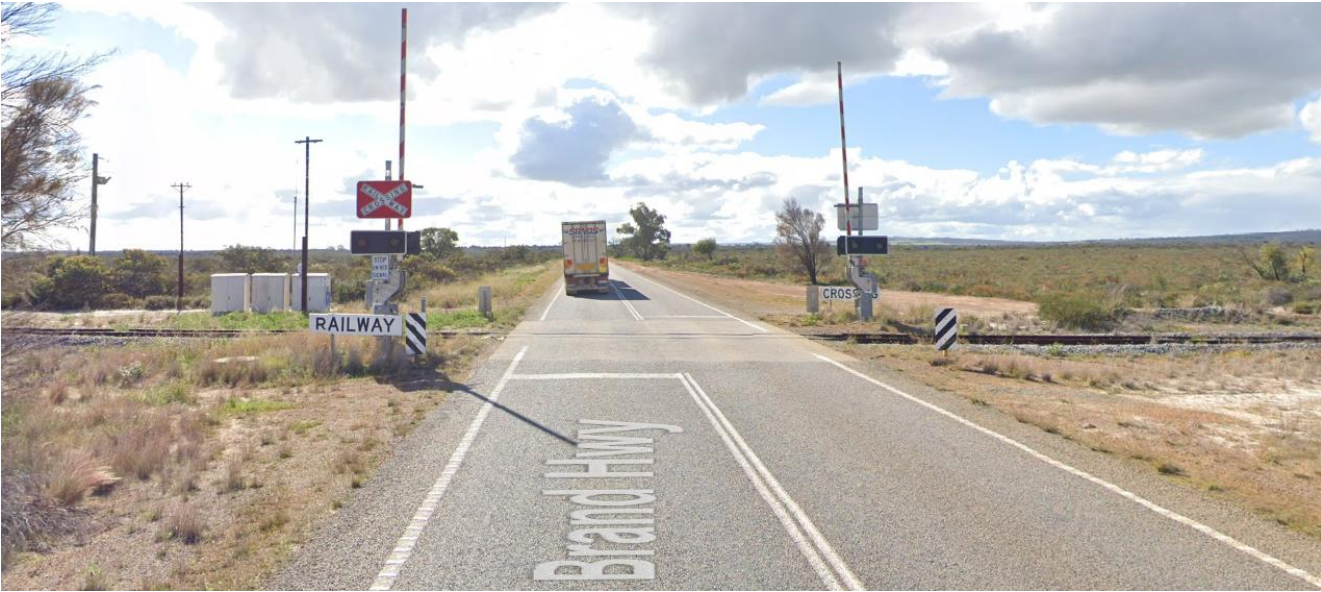
Figure 3-6: Existing Railway Level Crossing
