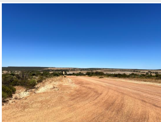
F6.3: Gate 1 Approach Looking Left (East)
