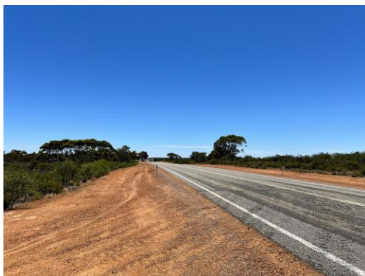
F8.3: Gate 3 Approach Looking Left (Northeast)
