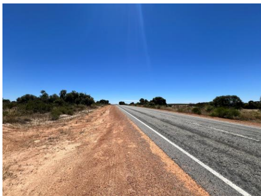
F19.3: Gate 14 Approach Looking Left (Northwest)
