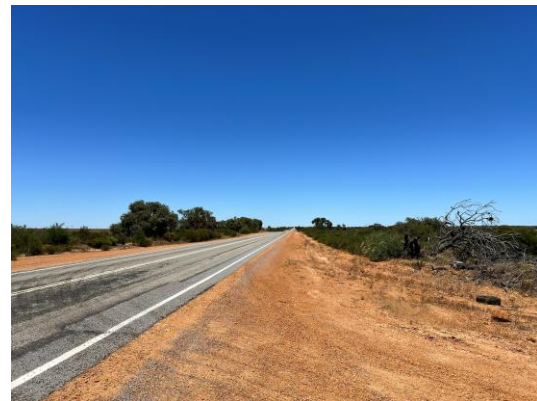
F8.4: Gate 3 Approach Looking Right (Southwest)
