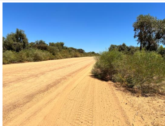
F21.4: Gate 16 Approach Facing Right (South)
