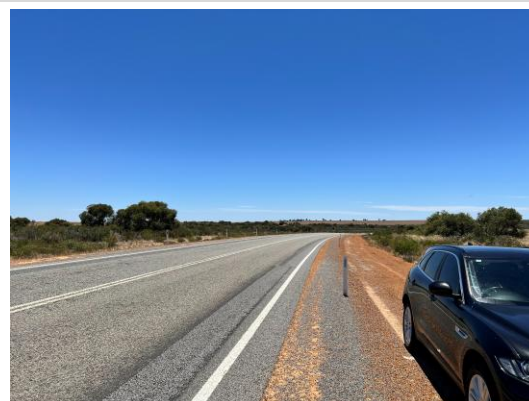
F10.4: Gate 5 Approach Looking Right (Southwest)
