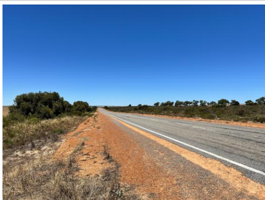
F9.3: Gate 4 Approach Looking Left (Northeast)
