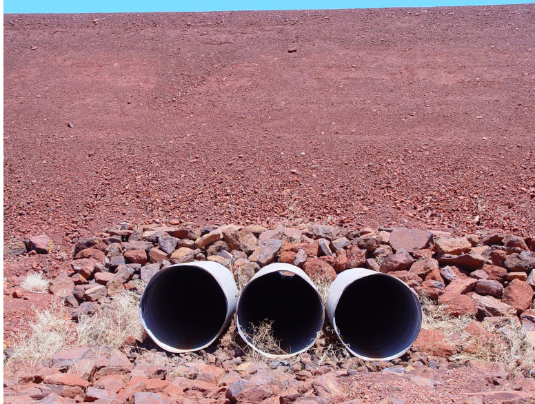
Figure 2.5 – Typical Culverts on the Mainline
