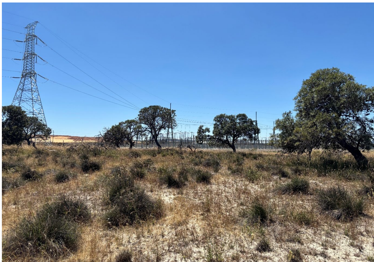
Plate 1: Cable connection vegetation
