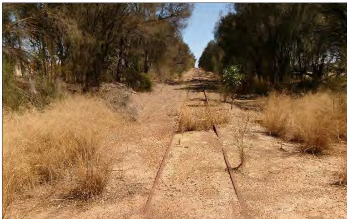
Figure 41: A disused railway line traversed by the 132kV underground transmission line corridor.
